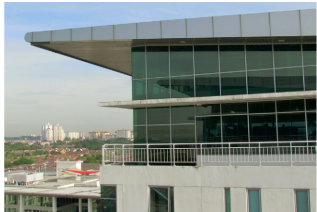
Figure 17.8f A major weakness in the design is the inadequate shading of many windows. Although the air-conditioned penthouses are enclosed by very low solar gain glazing, they are unbearably hot inside because of both solar and conduction gains. Instead, the penthouses should have had much less glass and extensive outdoor shading.
