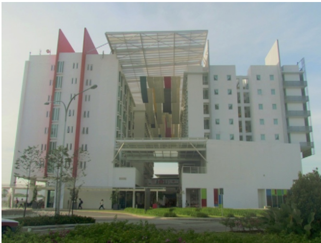
Figure 17.8e A shaded and protected atrium type of space is created between the two blocks of student housing. The windows facing this interior space are well shaded.
