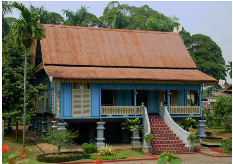
Figure 17.2e This traditional Indonesian house demonstrates many of the strategies appropriate in hot and humid climates. The house is raised on stilts both to get above the humidity and surface water on the ground and to raise the building to catch more wind. The high roof allows for stratification and good gable ventilation. The large covered porch provides shading for windows, walls, and an outdoor living space. To maximize natural ventilation, the windows are floor to ceiling and protected by louvered shutters.
