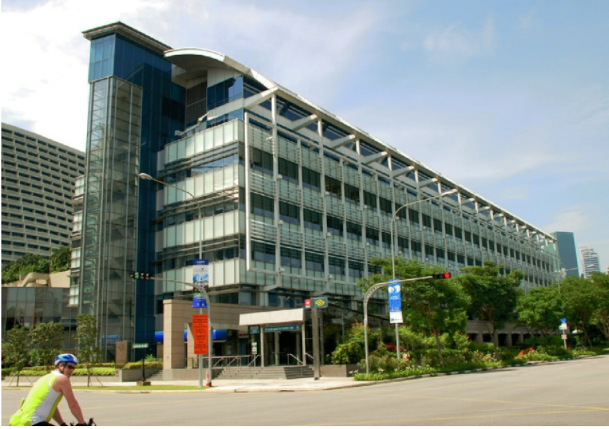
Figure 17.4d This building in Singapore seems to have gotten everything right: long axis running east–west, narrow rectangle to maximize daylighting, and exterior shading on the long facade. But what about the other long facade?
