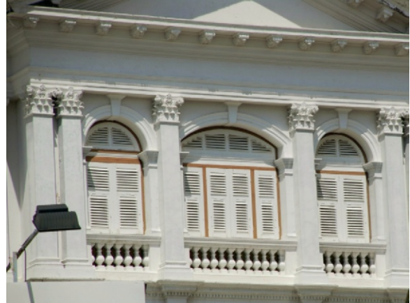
Figure 17.2k The design of this European-style building in Bangkok, Thailand, adjusted as much as possible to a climate alien to its origins by means of the extensive use of large windows protected by louvered shutters. Transplanting building styles that are appropriate for one climate to an alien and inappropriate climate is a phenomenon that runs throughout the history of architecture. Unfortunately, only in some cases are the styles modified either immediately or over time to fit the new climate. For example, Auburn University in the hot South is built in the English Georgian style more suitable for a mild cloudy climate.
