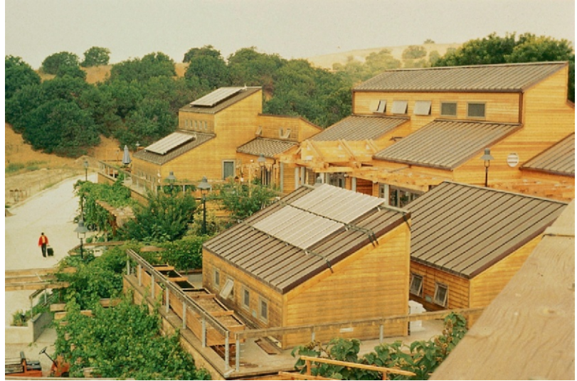
Figure 2.3b The Center for Regenerative Studies at Cal Poly Pomona was established to teach and explore how to restore the planet. The buildings are all oriented to the south, with few if any windows facing east or west. The roofs also face south to support active solar hot water collectors and future photovoltaic panels.
