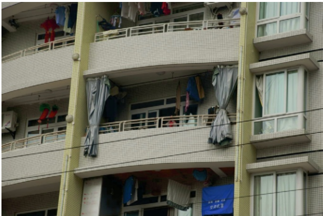
Figure 17.5 The smart condo owners in this Chongqing, China, apartment building added reflective curtains at the outer edge of their balconies to shade not only the windows but also the balcony.
