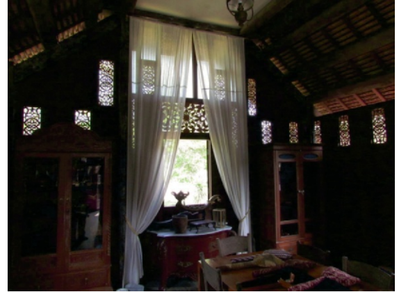
Figure 17.2h This traditional upper-class home in Malaysia maximizes natural ventilation while providing significant security through carved screens and windows with shutters. Note how the roof seems to float on the walls to further maximize natural ventilation.
