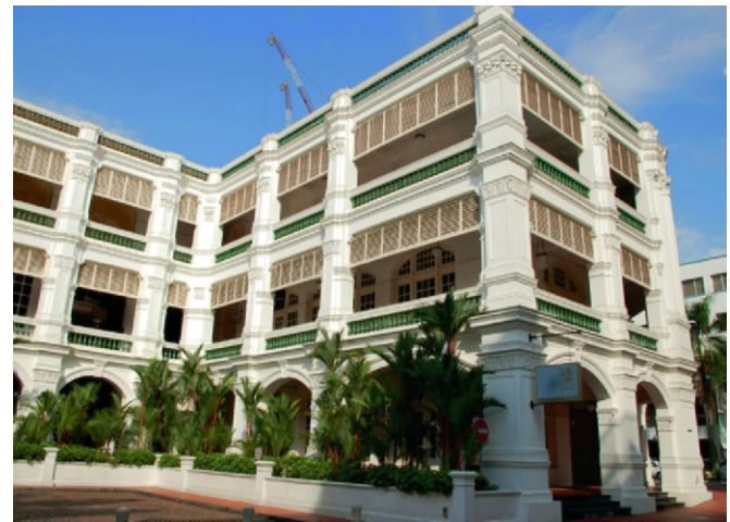
Figure 17.2l The Raffles Hotel in Singapore is an example of a European colonial building very well adapted to the local hot and humid climate. Not only are all of the rooms protected by exterior corridors, but also the low sun is blocked by louvered screens.
