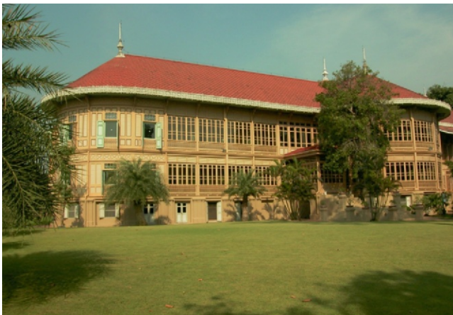
Figure 17.2j Lack of money was not the reason this royal palace in Bangkok, Thailand, was made of wood. Rather, it was the recognition that massive materials like stone and brick were inappropriate for promoting thermal comfort in a hot and humid climate. An abundance of beautiful carved wood screens under each window maximize ventilation.
