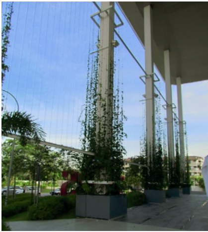
Figure 17.8c The east and west facades of the administrative building are protected by very large overhangs and vine trellises. This photo was taken shortly after the completion of construction. The vines should be doing great shading by now.
