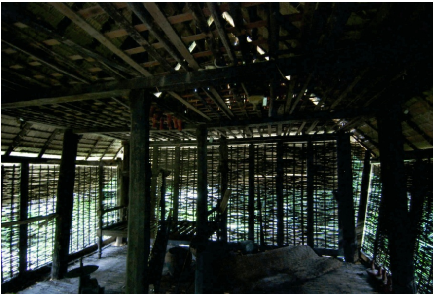
Figure 17.2g To maximize natural ventilation, this Southeast Asian rustic home has walls that are as porous as possible while still providing some security and privacy. Also note the gable vents that also allow light to enter.
