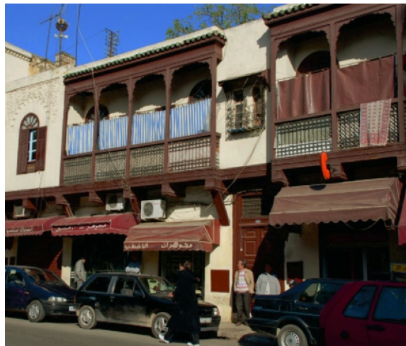
Figure 17.2b In hot climates, shade is the top priority for achieving thermal comfort. This street scene in modern Fez, Morocco, shows many of the strategies used: louvered shutters (far left), a small overhang (window in center), covered balconies, and outdoor curtains.
