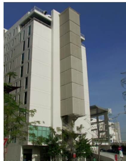
Figure 17.8b The classroom buildings at Taylor's University in Malaysia are properly designed by having their long axis running east–west and practically no windows on the short east and west facades. The outdoor projecting stairway is protected by a shade screen.
