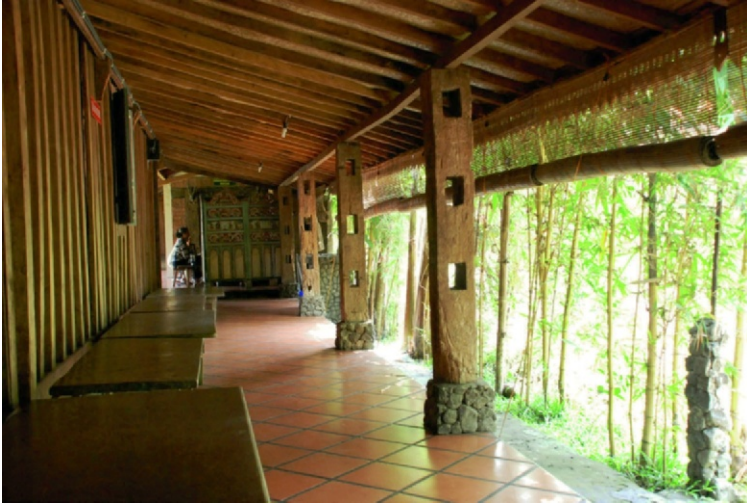
Figure 17.2f The low east and west sun make shading those orientations very difficult but especially necessary. A common solution was to have deep covered porches with roll-down bamboo curtains.
