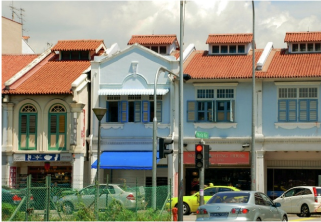
Figure 17.2i In the traditional urban Chinese building in hot and humid areas, the first floor was commercial and the second floor was residential. To maximize natural ventilation, the commercial activity was completely open to the street during the day, with awnings providing additional shade. Upstairs, large windows with louvered shutters allowed much natural ventilation at night and some during the day. The ventilation is greatly improved by the roof monitors, which operate through a combination of the stack effect, the Bernoulli effect, and the venturi effect (see Section 10.5 for an explanation of these).
