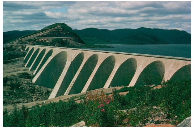
Figure 2.18k Hydroelectric dams produce pressure (head). Some also store water, and therefore energy, for later use.
