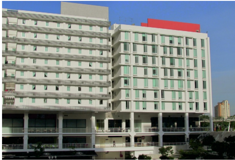
Figure 17.8d The student housing, unfortunately, was not oriented correctly and the east and west windows are not even shaded. But another good feature is that all of the buildings on this campus are connected by shaded passages.
