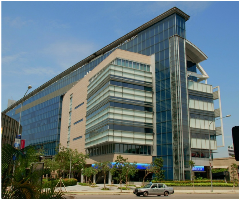
Figure 17.4e The other long facade of the building shown in Figure 17.4d looks as if it were the northern facade of a building in the northern temperate zone. However, Singapore is practically on the equator, so north and south facades should be the same.
