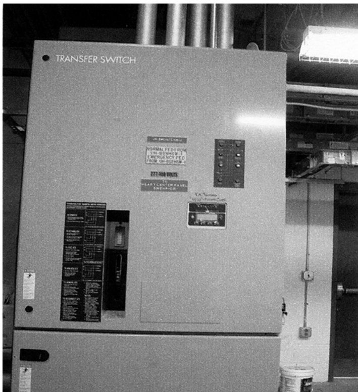
Figure 10-3 Emergency Load Transfer Switch
