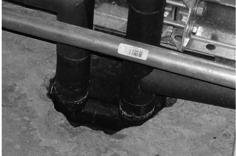
Figure 7-3 Core Bore of Concrete Floor to Install Condensate Trap
