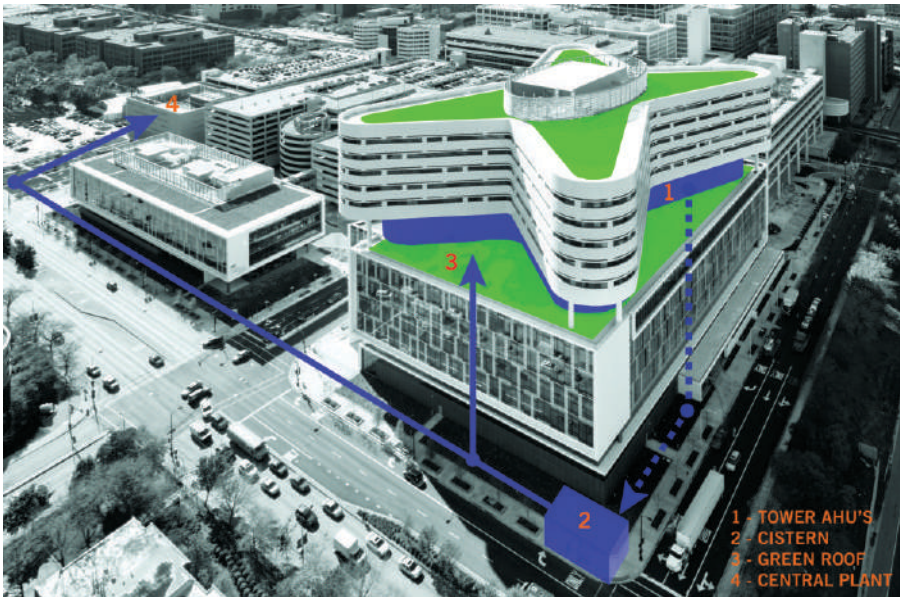
Green Features at Rush University Medical Center, Chicago, USA 1- Tower AHU's : 2-Cistern : 3-Green Roof : 4-Central Plant
