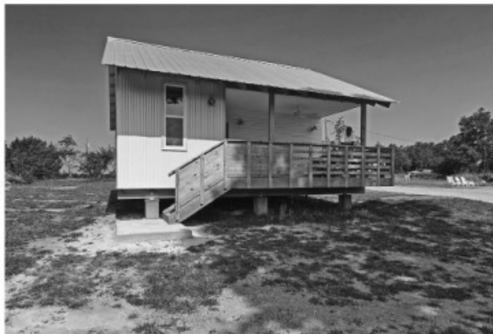
Figure 32.1 The Rural Studio at Auburn University has created a number of houses and public buildings for some of the most needy people in one of the poorest counties in the United States. Their design of a $20,000 house shows how good design can produce more value for less money than a mobile home.
