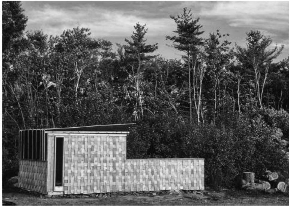
Figure 31.5 Richard Kroecker and his students at Dalhousie University have begun to look at materials in the modern waste stream, such as unused telephone books held in compression to form bearing walls of a “phone book building,” whose massive walls also provide ample insulation.
