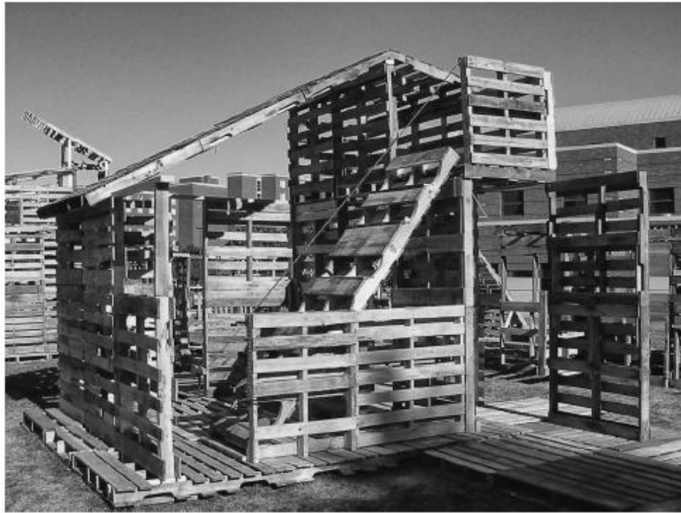
Figure 31.6 House with Sleeping Loft, Pallet Structure #3. Wes Janz's students at Ball State University, along with I-Beam Design, have developed ways to use the 1.9 million wood pallets destined for landfills in the United States for housing, drawing on the widespread use of pallets in squatter housing around the world.
